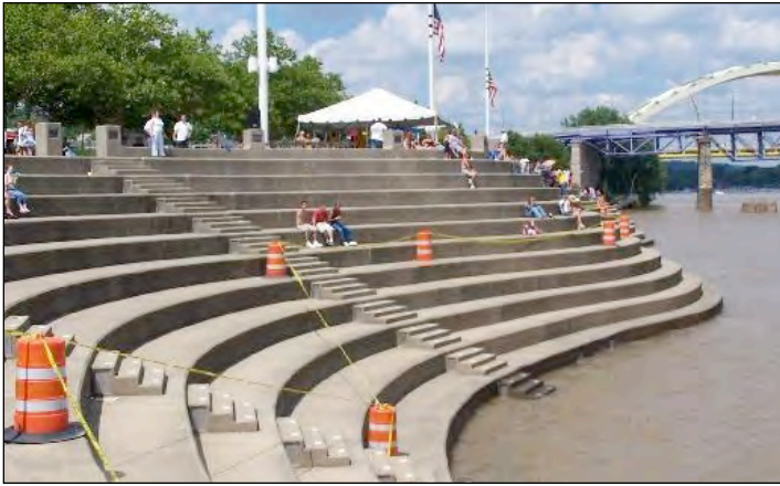
The Serpentine Wall at Yeatman's Park in Cincinnati is an undulating flood wall where the Ohio River laps against the bottom step. Serpentine walls are sometimes called crinkle crankle walls.
